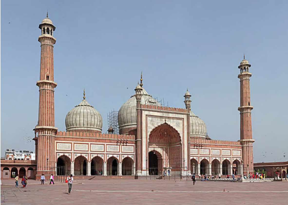
Jama Masjid in Delhi remains India's largest mosque and a classic example of the Mughal style of architecture.
