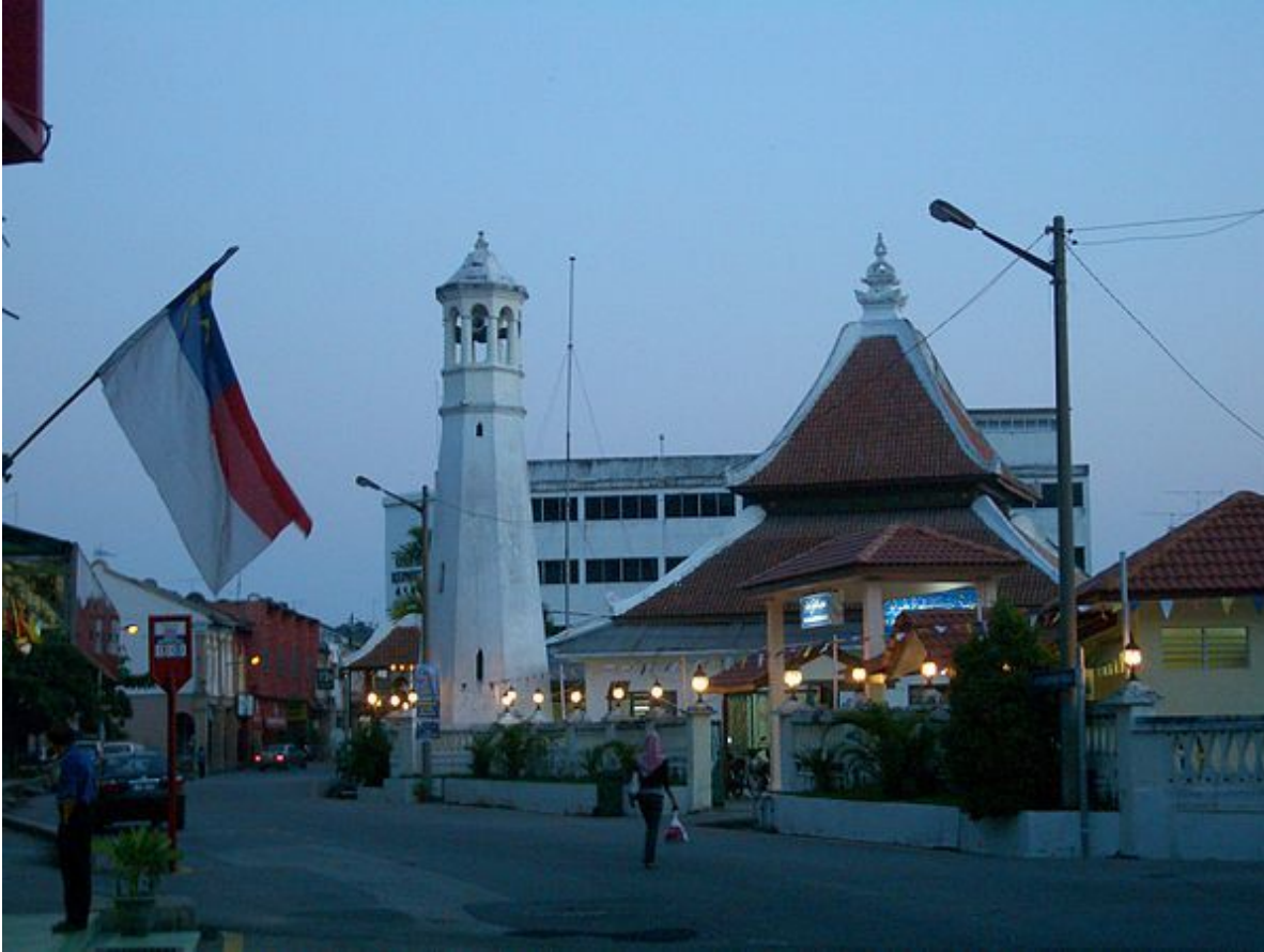
Kampung Hulu Mosque, the oldest mosque in Malaysia influenced by the Malay, Chinese and Hindu architecture.
